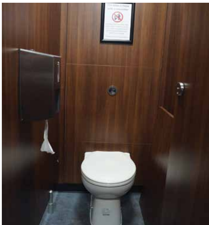
Access to the Sanicubic 2 XL for routine servicing and maintenance is simple thanks to the demountable panel on the right of this cubicle.
